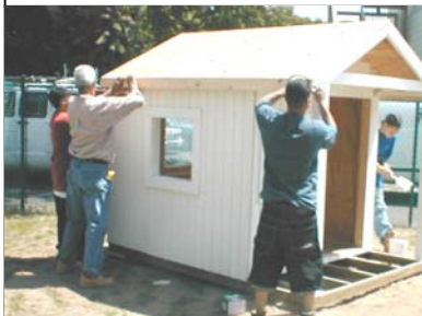
PA students building the new playhouse for CSR's daycare
