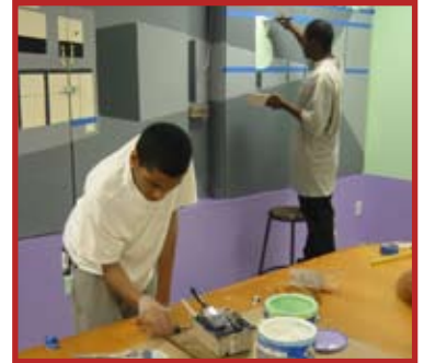
Interior work in progress at 504 Dudley St.
