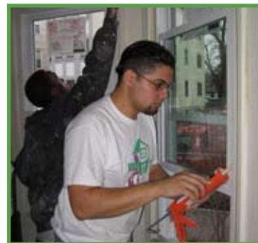
YouthBuild Boston trainees install windows.
